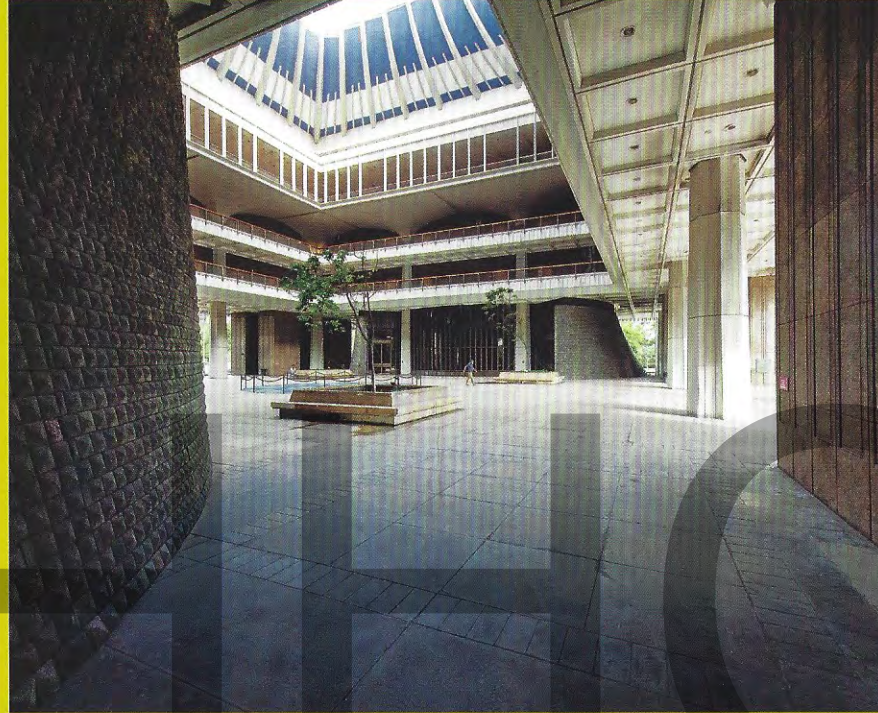
The rotunda, or open courtyard viewed from one of the four elevator cores which help support the building.
