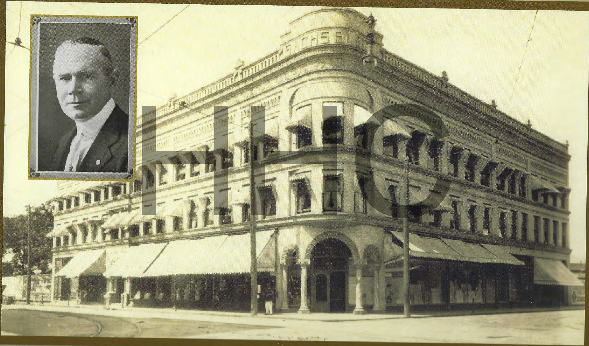
The formality of the three story, renaissance revival Century Block, built for N.S. Sachs at the mauka-'Ewa corner of Fort and Beretania streets, was relieved by its rounded corner accentuated by a triumphal arched entry. Seemingly ahead of its times, this mixed use building had seven stores on the ground floor, offices on the second, and housing on the third. The main hall to the upstairs had ample room for the parking of the lodgers' bicycles, which would earn the building extra LEED points in today's world.
