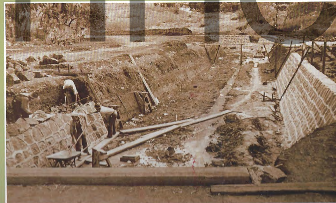
Woodlawn Drainage—Constructing retaining wall.
