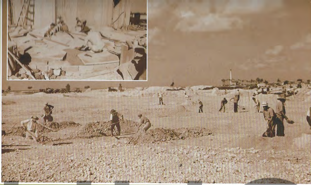
Ala Moana Park – Spreading Coral · (inset) Laying Sandstone Pavers at Entry
