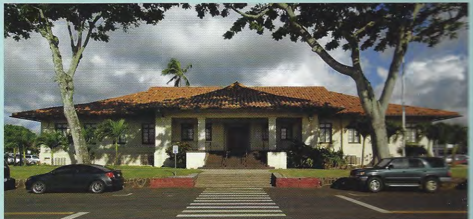
Lihue Circuit Court Building
