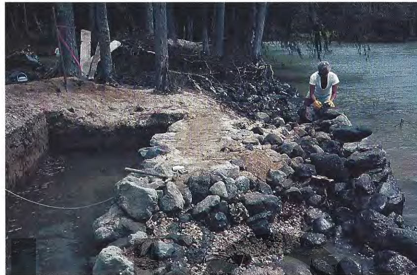
Wall restoration at Huilua Fishpond, O'ahu.
