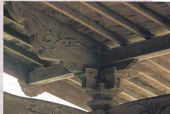
Elbow brackets supporting carved beams, Maui Jinsha Mission.
