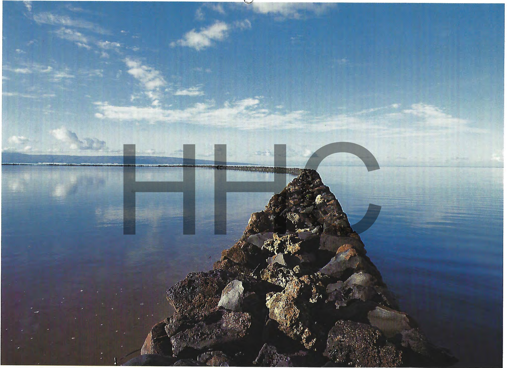
Kaloko'eli Fishpond, Kamiloloa, Moloka'i, Hawai'i Register of Historic Places. More than 300 fishponds, small and large, once lined the Islands' coastlines. They were built for the chiefs (ali'i) with walls of coral, stone or both. Gates with grills kept fish in and allowed circulation of fresh seawater. This type of aquaculture was unique to Hawai'i.
